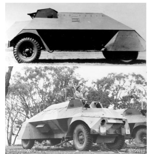
Top: Prototype Rover Mark I: Above, production Rover Mark I, serials for the Mk I ran from 77501 to 77538 plus 77553 and 77554. (Photos: Top: Author's collection. Above AWM)
