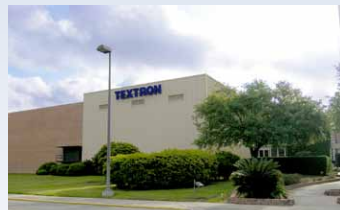
TM&LS Administrative and Engineering offices, Slidell, LA
