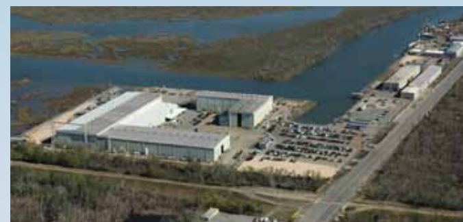
TM&LS New Orleans shipyard/armored vehicle fabrication facility
