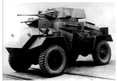
Above: Two views of an early Humber Armored Car Mk I is the 15mm and 7.92mm BESAs instead of the twin Vickers machine guns mounted by the Armored Car Guy Mk I.
