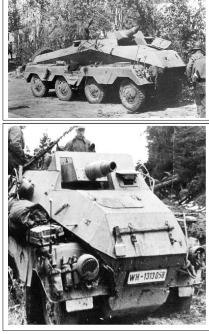
**Remarks**: 199 SdKfz 233 (7.5cm) vehicles were built new or converted from existing radio and reconnaissance vehicles with the first introduced to combat units in October of 1942. A fairly mobile vehicle, the KwK 37 L/24 cannon besides smoke and high explosive four anti-tank rounds were also available. The high explosive round had a range of 4923 yds (4500 m) while at 1094 yds (1000 m) the cannon was able to defeat from 1.4 in (35 mm) to 3.9 in (100 mm) of armor plate at 30 degrees angle.
