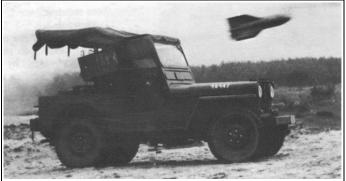
Above: As the vehicles left over from WWII began to wear out, Belgium acquired some new build, Willys M38s. The above vehicle is fitted with French built ENTAC anti-tank missiles.
