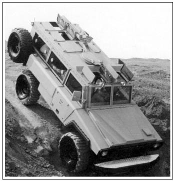
Drive, 4x4. Armor, protected up to 7.62mm or 14 kgs of TNT. NBC Protection, No. *Armament:* (1) .50 cal HMG. Elevation, manual. Traverse, manual. *Capacity:* Fuel, diesel.
