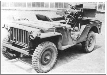
Above: Carr, Wpns, 4x4, Carriage, Motor, 37mm Gun, T2. Remarks: Based on the "Bantam" 1/4-ton Truck, Reconnaissance. A 37mm anti-tank gun with shield was mounted at the rear of the striped down chassis. Curved rear fenders were fitted at first, but these were later removed. T2 had gun firing to the rear.
