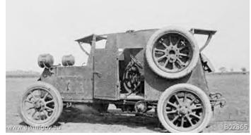
built armored cars produced in Australia on donated car chassis circa 1915. The bare chassis was supplied to the Vulcan Iron Works which applied the armored body. The Mercedes had a full rotating turret and was at armed with a .30 caliber Colt machine gun. Usage: Australian Army in the Middle East. Manufacturer: Mercedes/Vulcan Iron Works.
