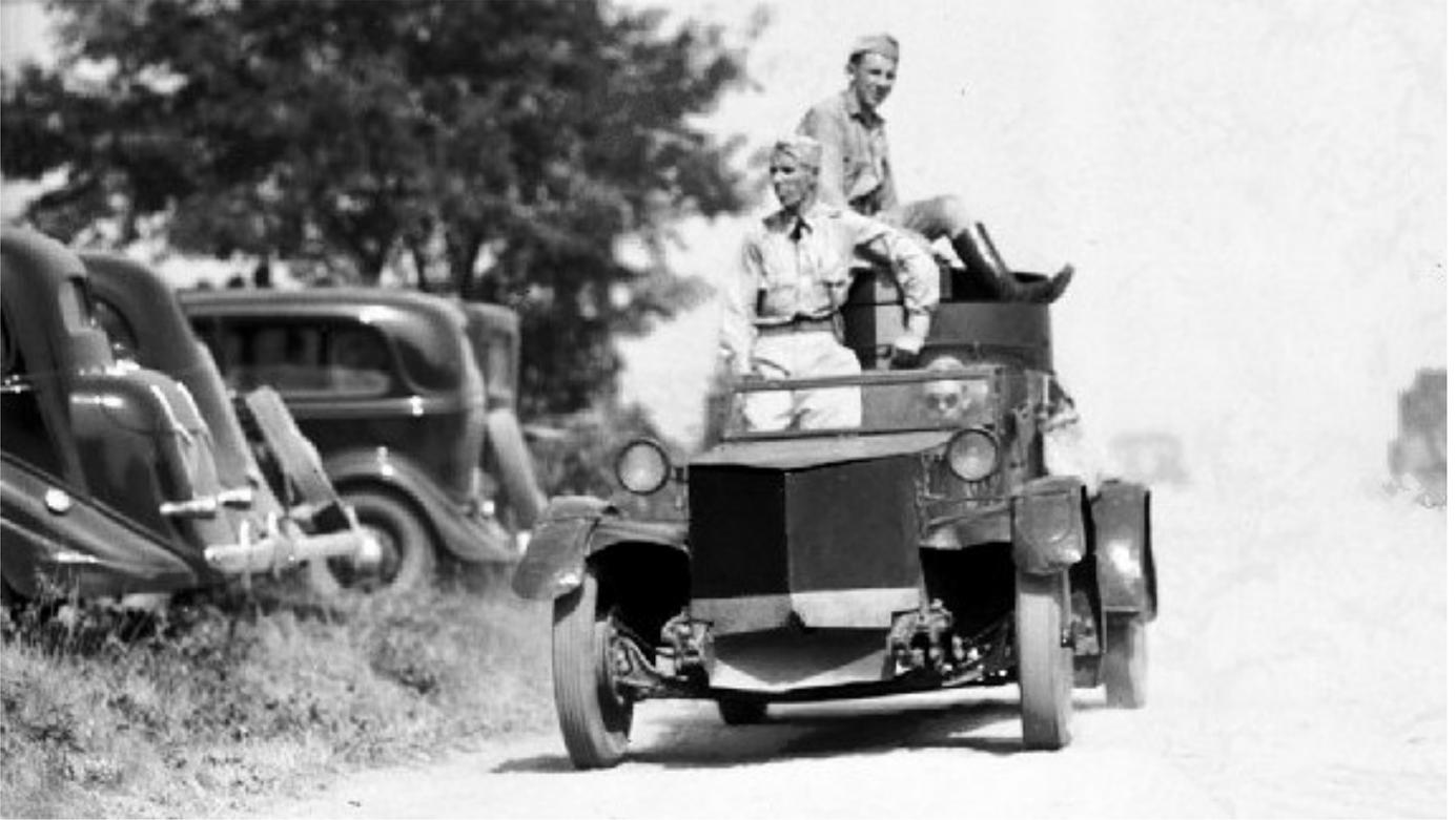
**1930 T9 Armored Car W-1317.** The T9 was built on a Plymouth chassis and had heavy spoked wheels. The armor plate at the bottom was cut off square, but the rear portion of the armor was lower than the front (opposite of the T8).
