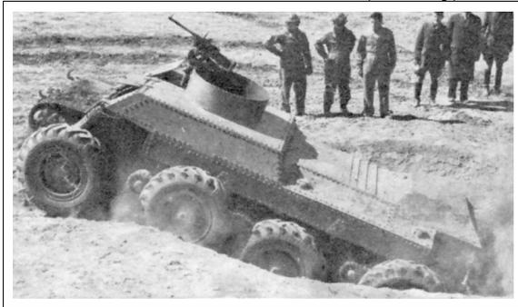
**Remarks:** A private venture by the Trackless Tank Corporation, the vehicle was tested by the Armored Board for use as an armored car, rather than as a tank. Chain drive was used to the last three axles, the front axle being used for steering. While no orders were awarded for the Trackless Tank, it did directly lead to the T13 Armored Car.
