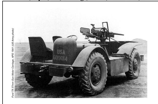
**Remarks:** Ford, "Swamp Buggy", 37mm gun fired forward, 4x4, circa 1941. Fifteen vehicles were built and tested. Project ended in favor of the 37mm Gun Motor Carriage, M6. Two vehicles were later modified into the Observation Post Tender T1 & T2 and at least a few vehicles were bought by the Dutch for the Neatherlands East Indies.
