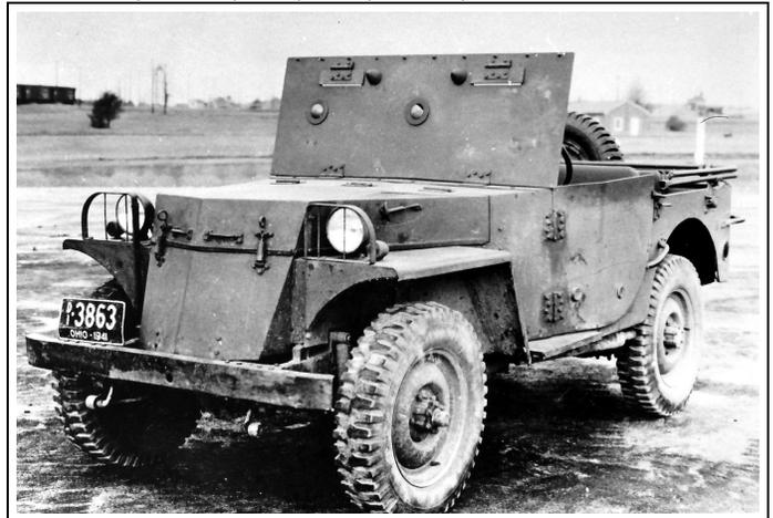
This vehicle was the Scout Car T25 re-modified with 1/4" armor on the frontal surfaces and a .30 cal. LMG in a ball mount in the windshield. Reopened in June of 1942, the vehicle was still too heavy and the project was closed again in 1943.
