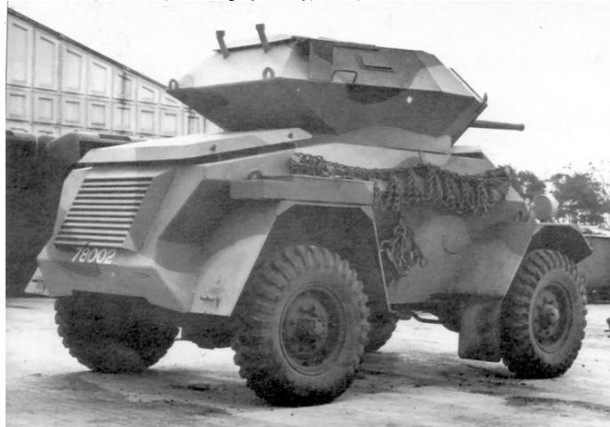
**Remarks:** Used the same General Motors of Canada (CMP) chassis as the Canadian, Fox, 4x4 armored car. Between one and four pilot vehicles were completed, but no series production was started.
