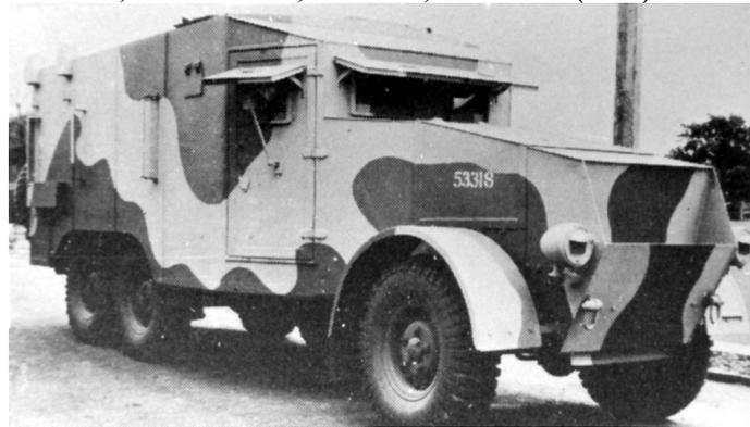
**Remarks:** 6x6 command vehicle based on the Truck 3-ton, 6x6, Ford/Marmon-Herrington. Double doors and spare tire at the rear. Limited production run, used only by Australia.
